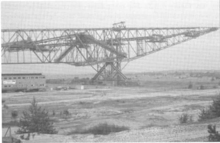
Figure 7.8-6: Recently, the protection of historical landscapes has been extended to interesting industrial areas: A conveyor bridge beat up in the closed lignite opencast mine "Bergheide" in the Lower Lusatian lignite mining region (Photo: O. Bastian 2001)
